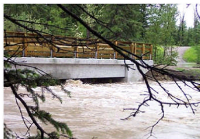
New 37 th St. Bridge, Calgary, Alberta. June 2005 flood. Source. Calgary Herald.
